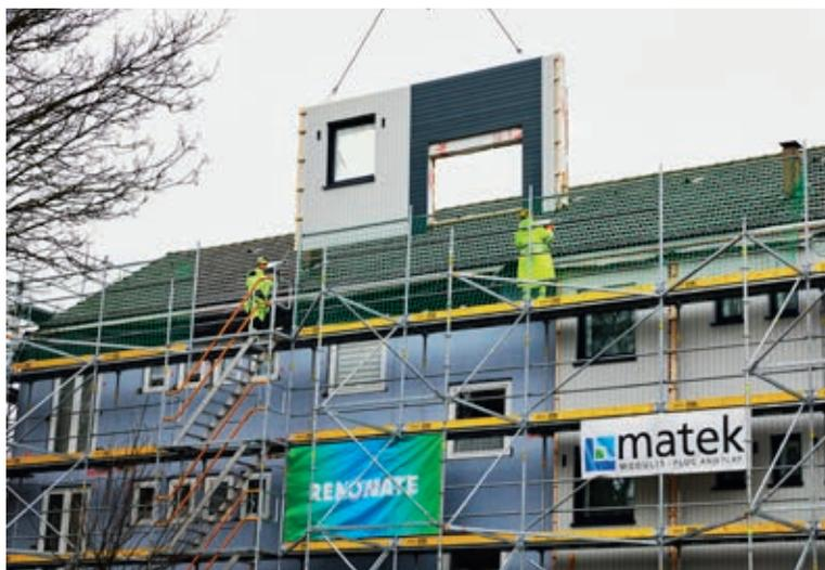
Assembly of a serially prefabricated façade in the English settlement in Soest.
