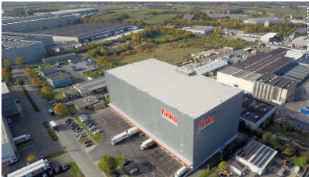
Finke Hochregallager Paderborn / Finke High bay warehouse Paderborn
