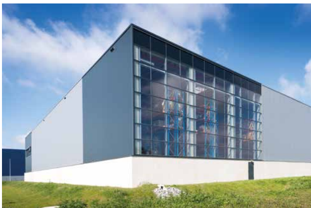
GLASS FRONT OF THE MÖMAX LOGISTICS CENTRE BERLIN (Source: BREMER)
