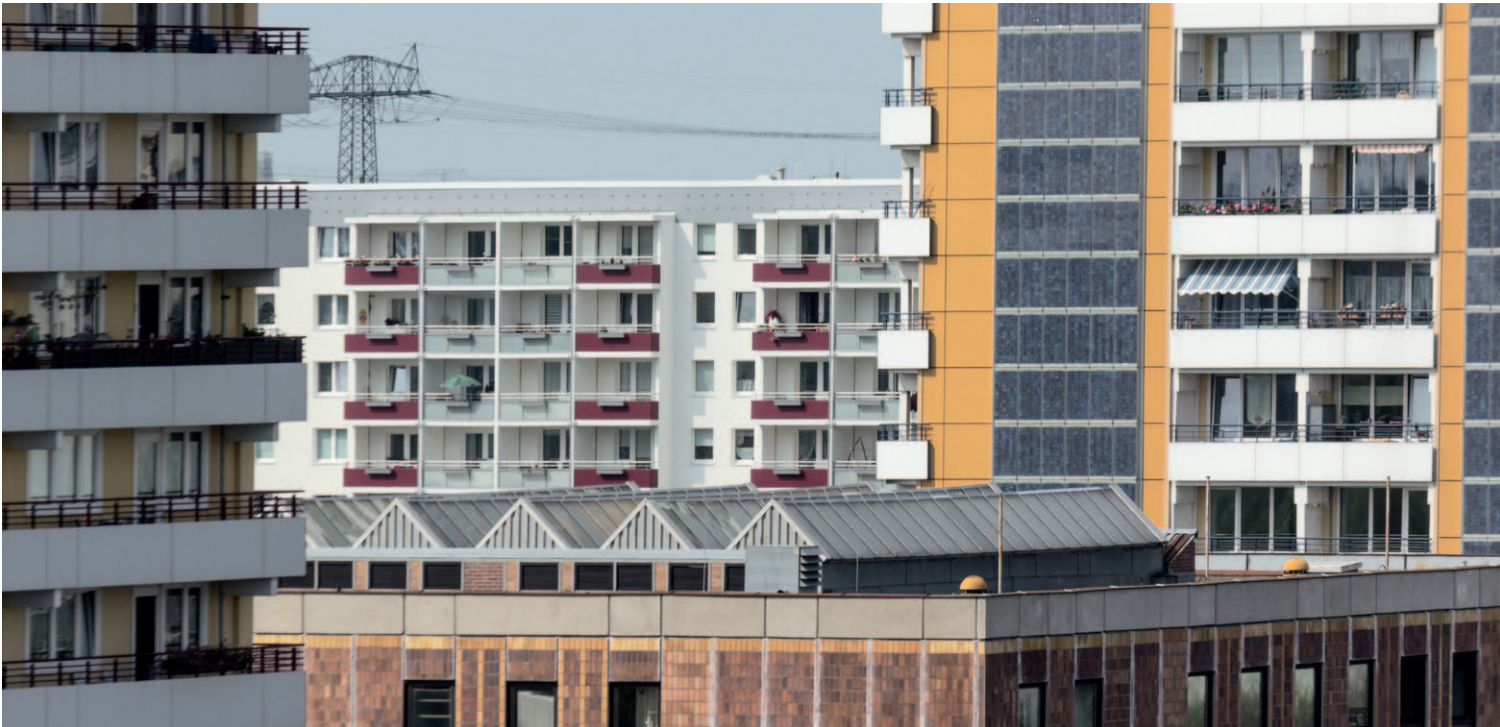
Affordable and practical: Renovated apartment buildings and a commercial building in one of the service centres of a GDR-era development in Marzahn-Hellersdorf
