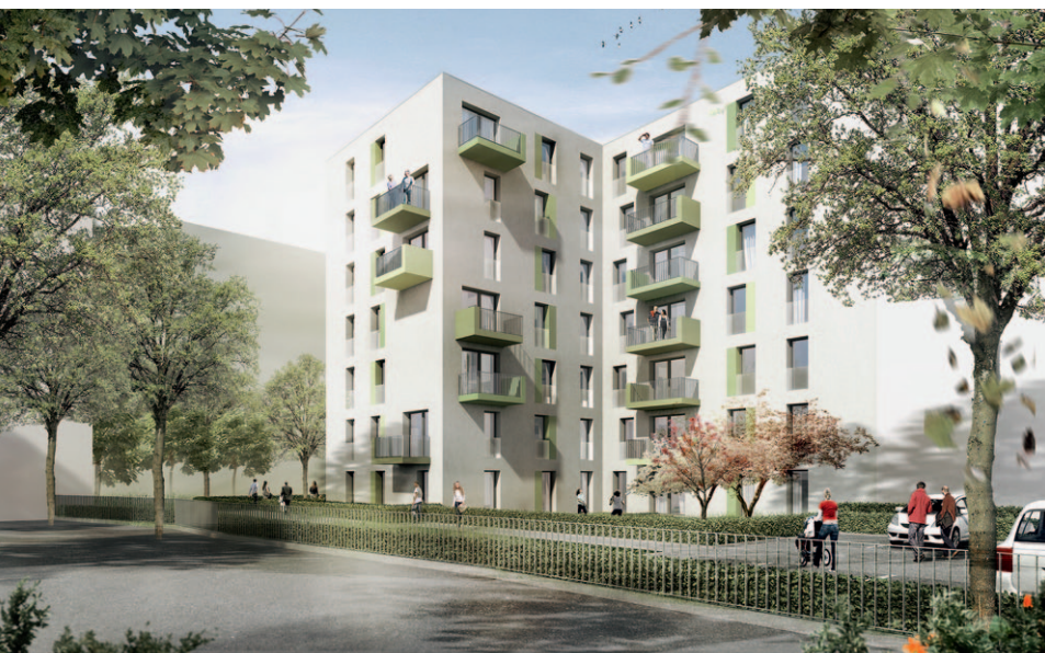
WBM (Wohnungsbaugesellschaft Berlin-Mitte mbH) is building 89 new apartments in Eckertstraße near Karl-Marx-Allee in Berlin-Friedrichshain
